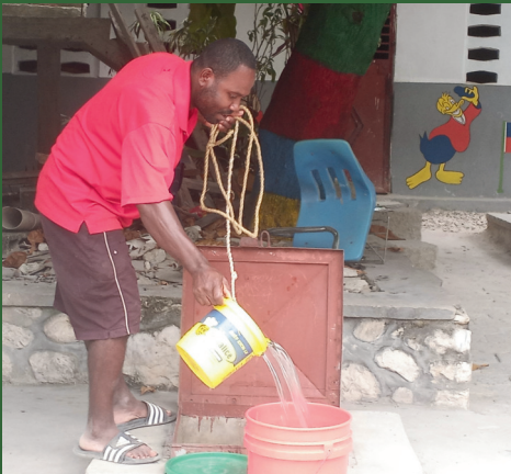
Underground tank for rain collection, storage, and retrieval
